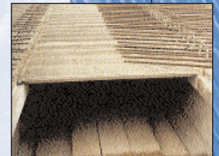
Bridgedeck Formwork - Europe
