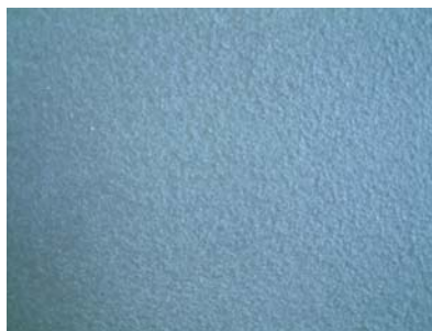
No Air Holes or Slump Lines
